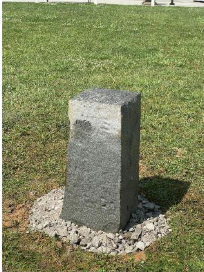
Fig. 14: Stone Monument in place and trimmed out.
