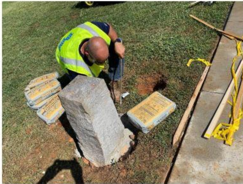
Fig. 13: Matt Rogers, PE, preparing to place concrete around the stone.
