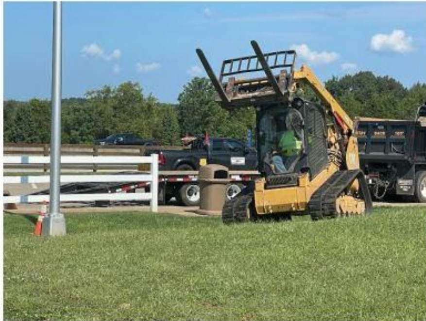
Fig. 11: Scotty's Contracting and Stone skid steer machine arriving on site.
