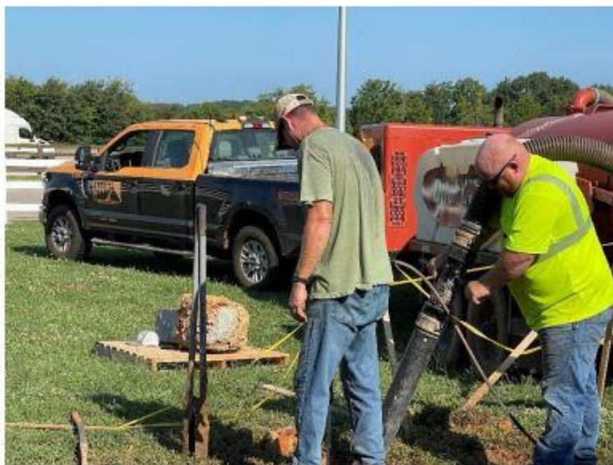
Fig. 10: Scotty’s Contracting and Stone Personnel performing the hydro-excavating of the holes.
